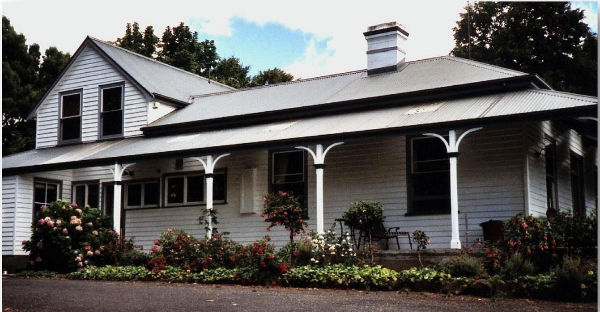
Poimena in 2005, The two-story section is a more recent addition.
